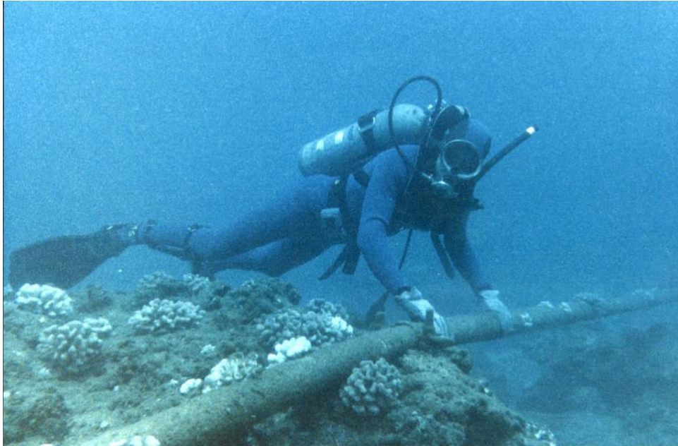
FIGURE 3: “Diver Checking Underwater Protection of Cable” 58
