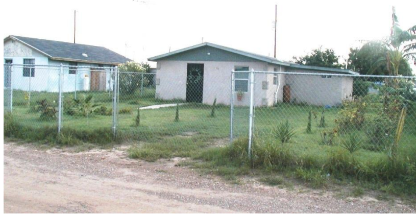
Figure 1.3. Stick frame housing (modular) on slab, Cameron Park, Cameron County
