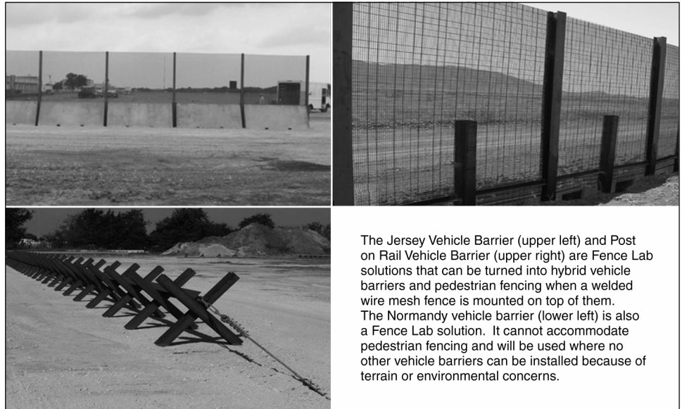
Figure 6: Vehicle Barriers and Fencing Developed by Fence Lab That Meet Performance Requirements and Are Included in SBInet’s “Toolbox” of Approved Fences and Barriers.
