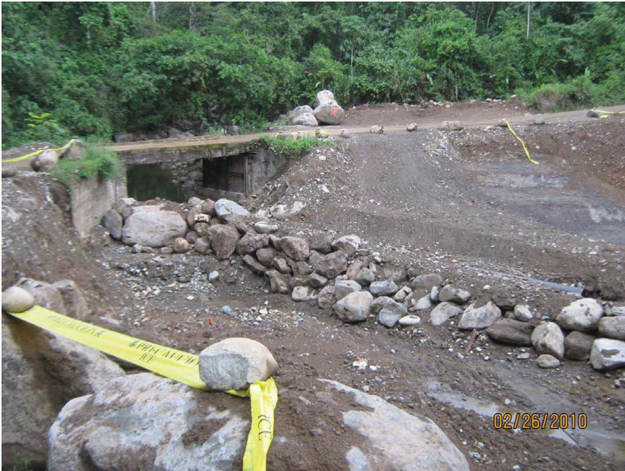
Figure 9. Construction in (and destruction of) the Veraguas stream. The stream, which runs through a ravine, is of great cultural importance and serves as an integral source of recreation and sustenance for the community. See also Figure 2. 165
