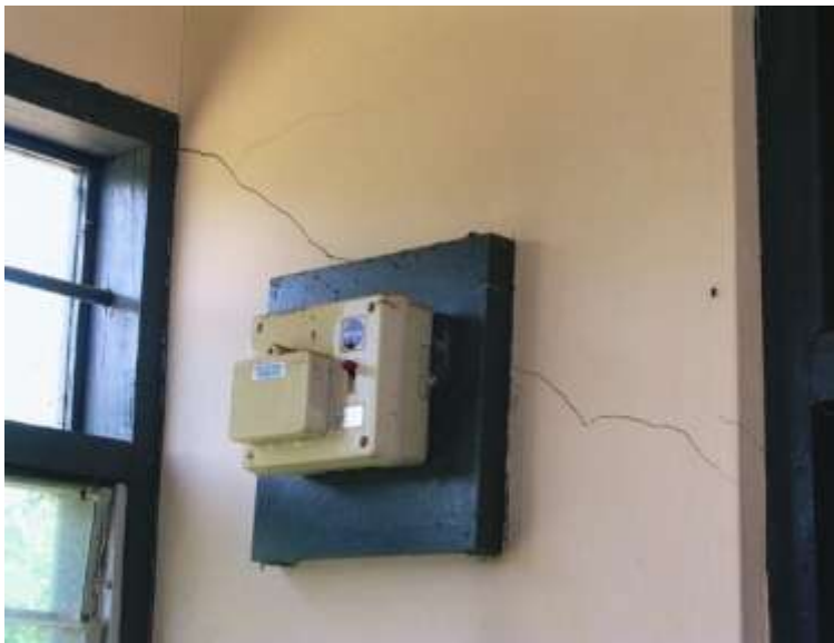
Cracks in the post office, which is much sturdier than many of the community members' homes, in Prestea due to mining blasting activity.
