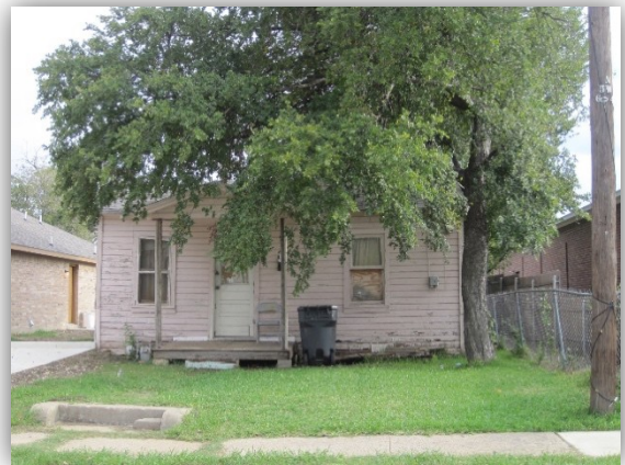
Abandoned home in Dallas.
