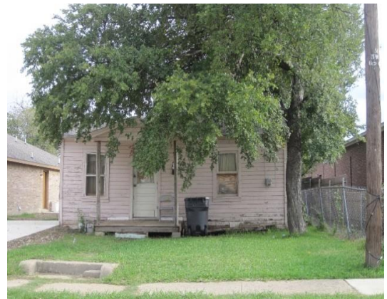
Abandoned home in Dallas
