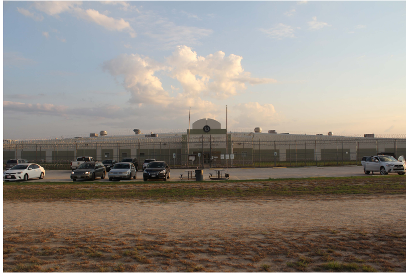
Figure 4. La Salle County Regional Detention Center, Encinal, Texas. The private prison corporation, Emerald Companies, broke ground on this female and male detention facility in 2002. Today it houses migrants awaiting trial and civilian convicts. Photographed by C. J. Alvarez
